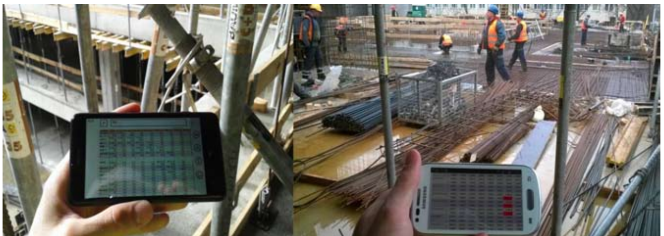
Figure 4. Smartphone application of Mobile Earned Value Monitoring System (MEVMS) on a construction site. Nokia Lumia 625 (left), Samsung S3 Mini (right).
