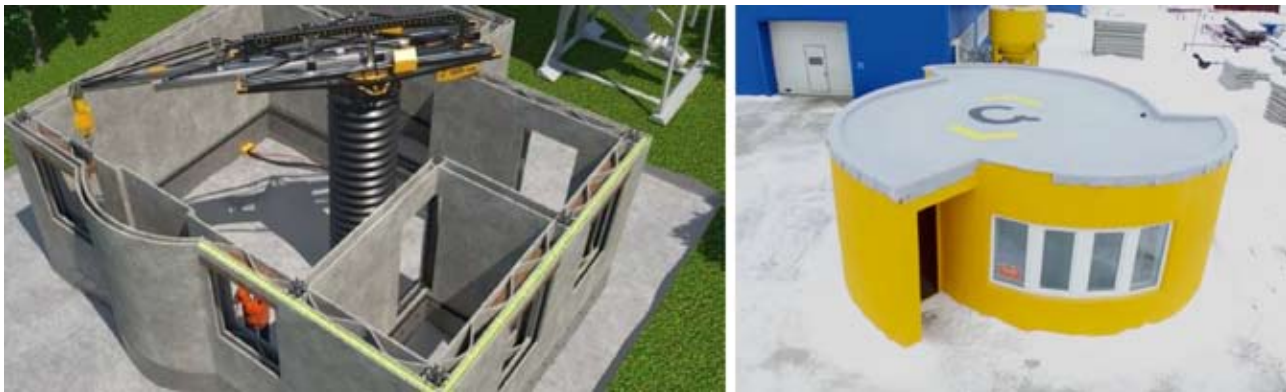
Figure 3. Apis Cor House 3D Printing
