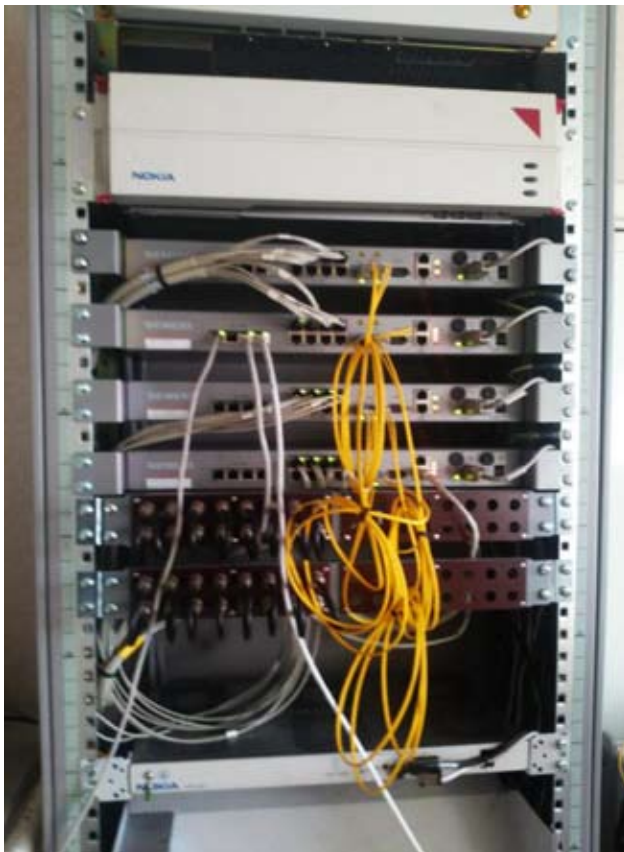
Figure 5. SIEMENS SURPASS hiT7020 – 4 multiplexers with subscriber system connections are connected to the ring via optical STM-1 interfaces.
